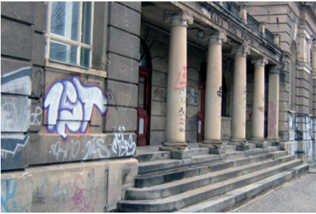
Fig. 1: Graffiti sprayed on protected buildings.
